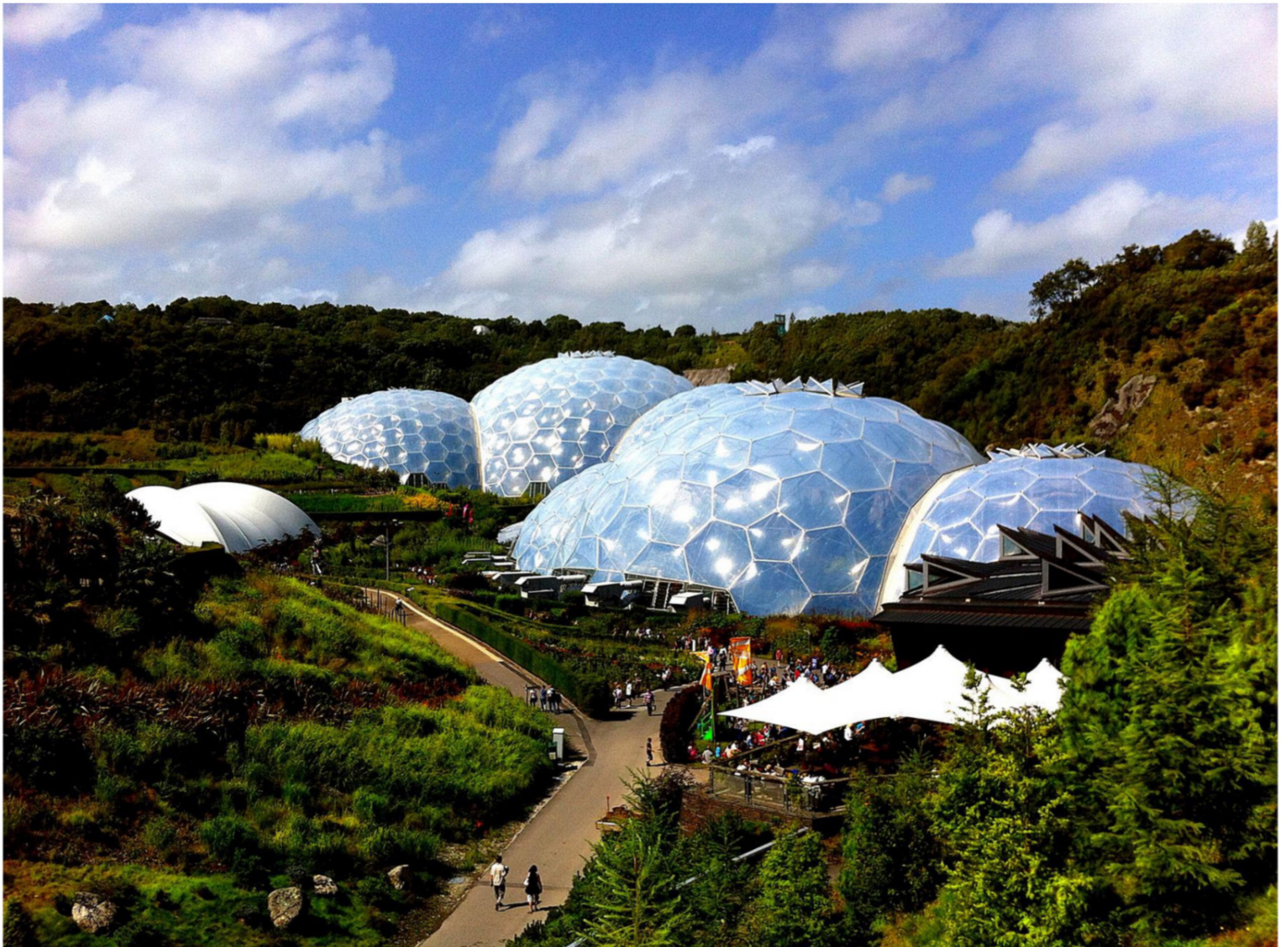
The impressive Eden Project in Cornwall, with its iconic domes by Grimshaw that host ecosystems from around the world.
