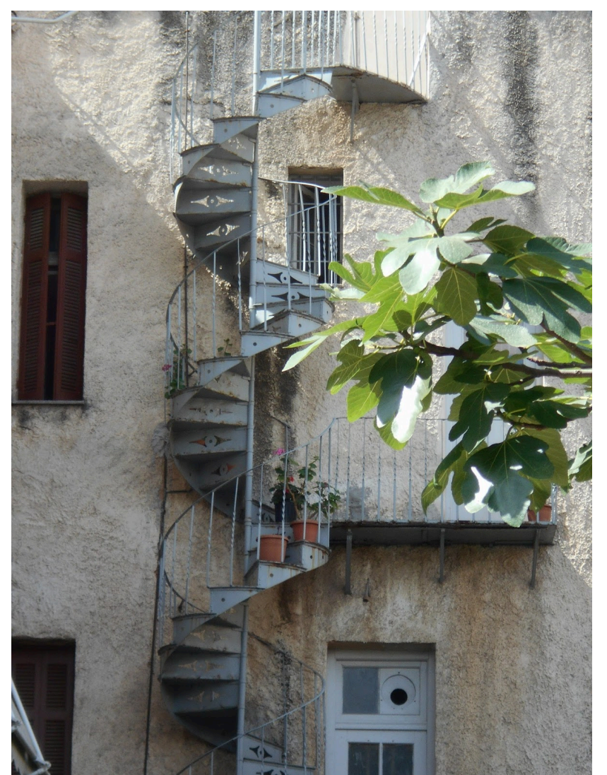
Service staircase leading to the washroom Athens / Plaka 1958
